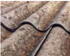
Chapas de asbesto-cemento
